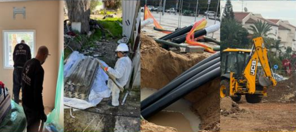
Early Utilities Relocation
